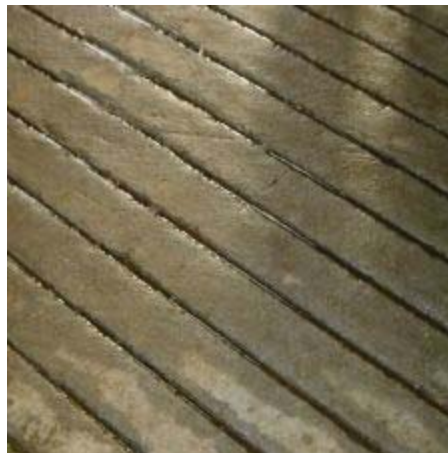
Figure 9b Grooves in concrete to prevent slipping of animals
