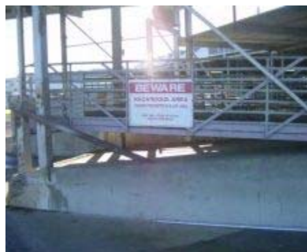
Figure 3 Ramp which can be adjusted to accommodate lorry
