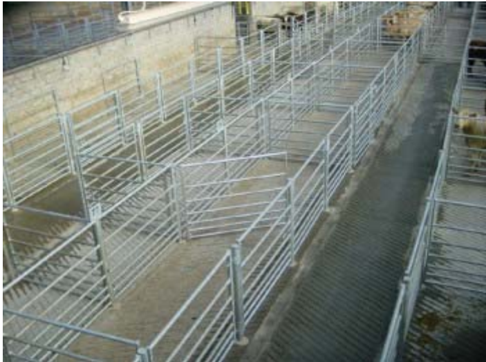
Figure 16 Pens which can be opened in sequence to make a straight passage
