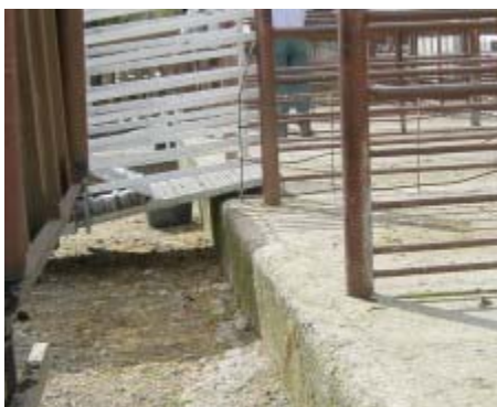
Figure 2 Unloading bay with raised step
